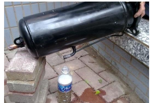
Figure 6-2.5: Draining oil from a compressor
