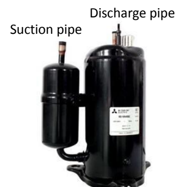
Figure 6-2.5: Compressor piping
