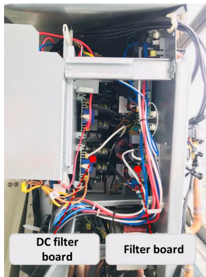
Figure 5-1.3: 14/16HP rear view of electric control box
